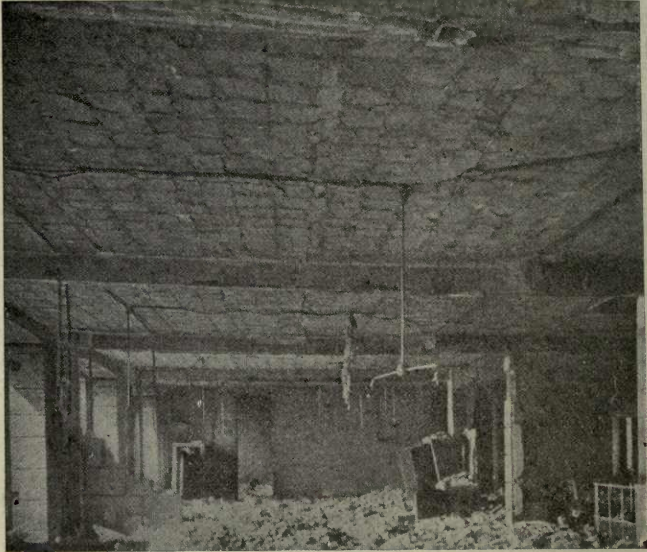
FIG. 39. — Interior of Herald Building, Baltimore Fire.
